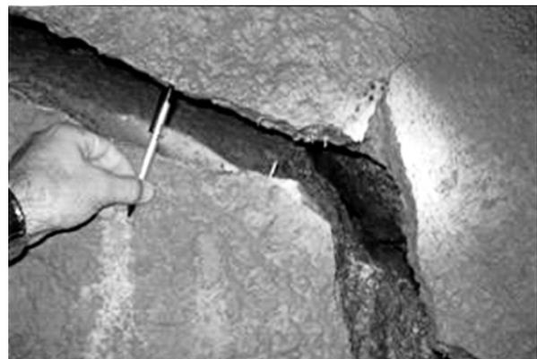
Figure 1. Rock fracture opened by hydrofracturing in a pressure tunnel with support only of shotcrete.
