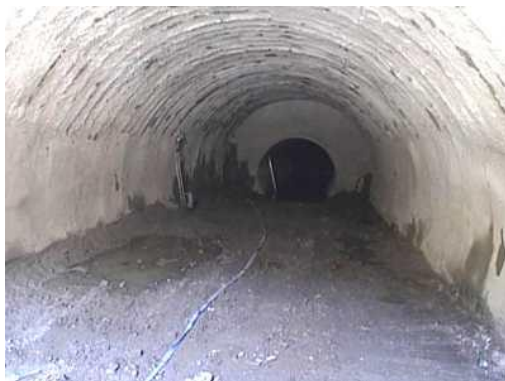
Figure 11. Aspect of the Northern part of the tunnel station the day before its collapse, with no fissures or any sign of instability problem.
